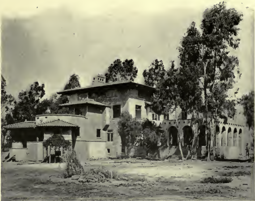
RESIDENCE AT LOS ANGELES, CAL.
